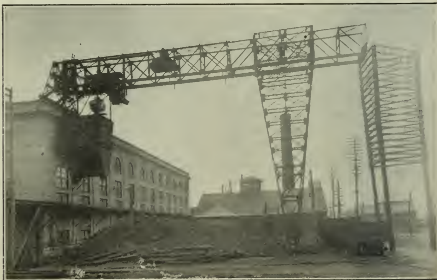
FIG. 2. COAL HANDLING FROM CAR TO PLANT
